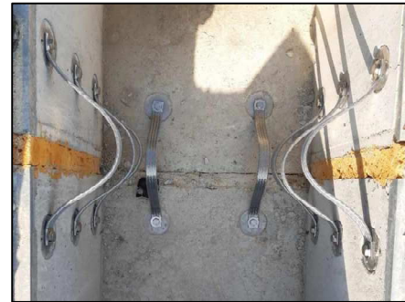
Fig. 3. Interconnection of two sections of the concrete duct.
